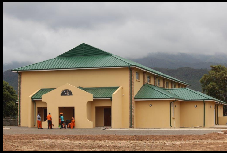
Moshate Community Hall
